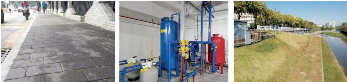
图 6 透水铺装、雨水回用系统和植被缓冲带(布吉河)效果图 Fig.6 Effect pictures of permeable pavement, rainwater reuse system and vegetation buffer strips (Buji River)
