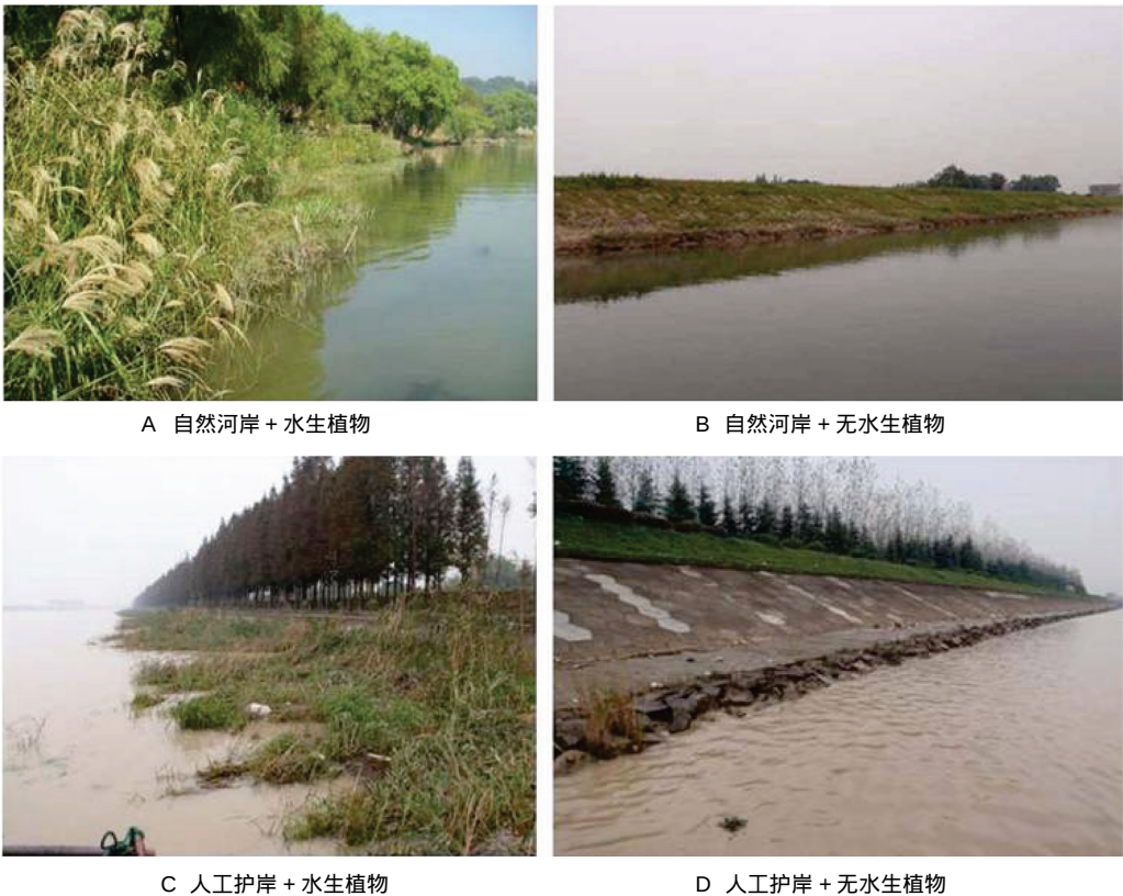
图 3 东苕溪中下游 4 种河岸类型 Fig. 3 The four bank types in the middle-lower reaches in the East Tiaoxi River
